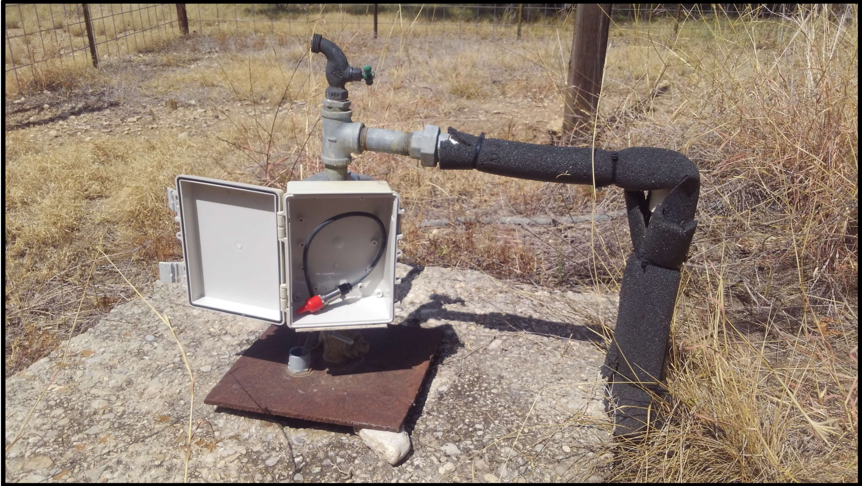
Direct Read Cable Installation – Exempt Well
