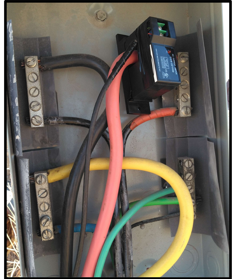
Current Switch Installation
